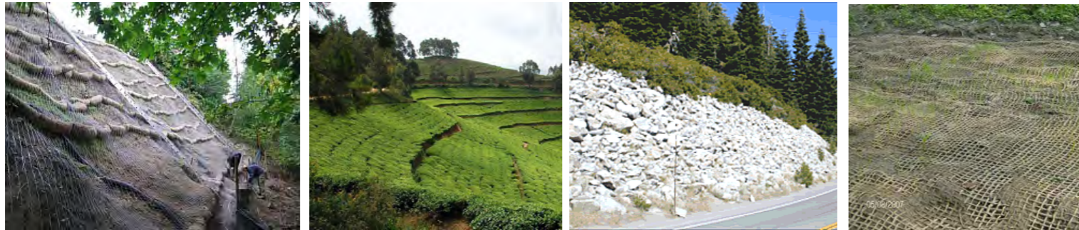
Use appropriate slope management techniques like rock slope protection, Slope Roughening, Terracing, and Rounding, mulching, erosion control mats etc for different slope categories Fig.7.24 Slope stabilization & erosion control techniques
