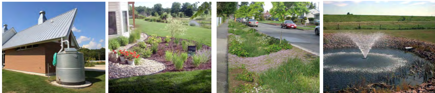
Use appropriate stormwater management techniques from unit to neighborhood level before it gets discharged into natural drains and wetlands. Like rainwater collection from rooftop, rain gardens, bioswales, retention ponds etc.
