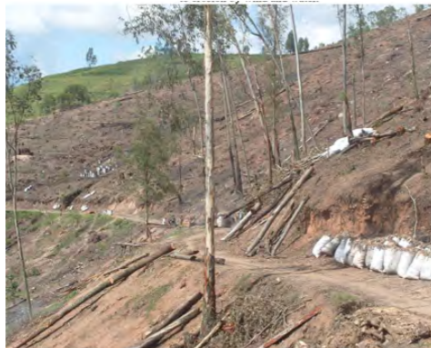
Heavy soil erosion along the steep slopes because of the forest plantation removal
