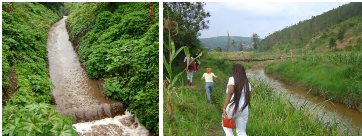
Propose vegetative buffer along natural drains to control soil erosion and allow habitat flow Use environmental buffers along the natural drains as park Fig.7.25 Watershed and stormwater management techniques
