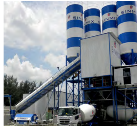
Construction Industry, Small factory and Dry Port
